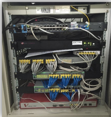
Server Installation / Maintenance
